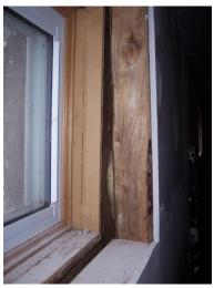
Picture 1: Gap where air can get behind basement insulation and cause mold growth.
